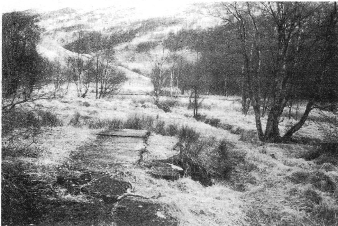
Looking over the base of a Nissen hut up river towards the dam
