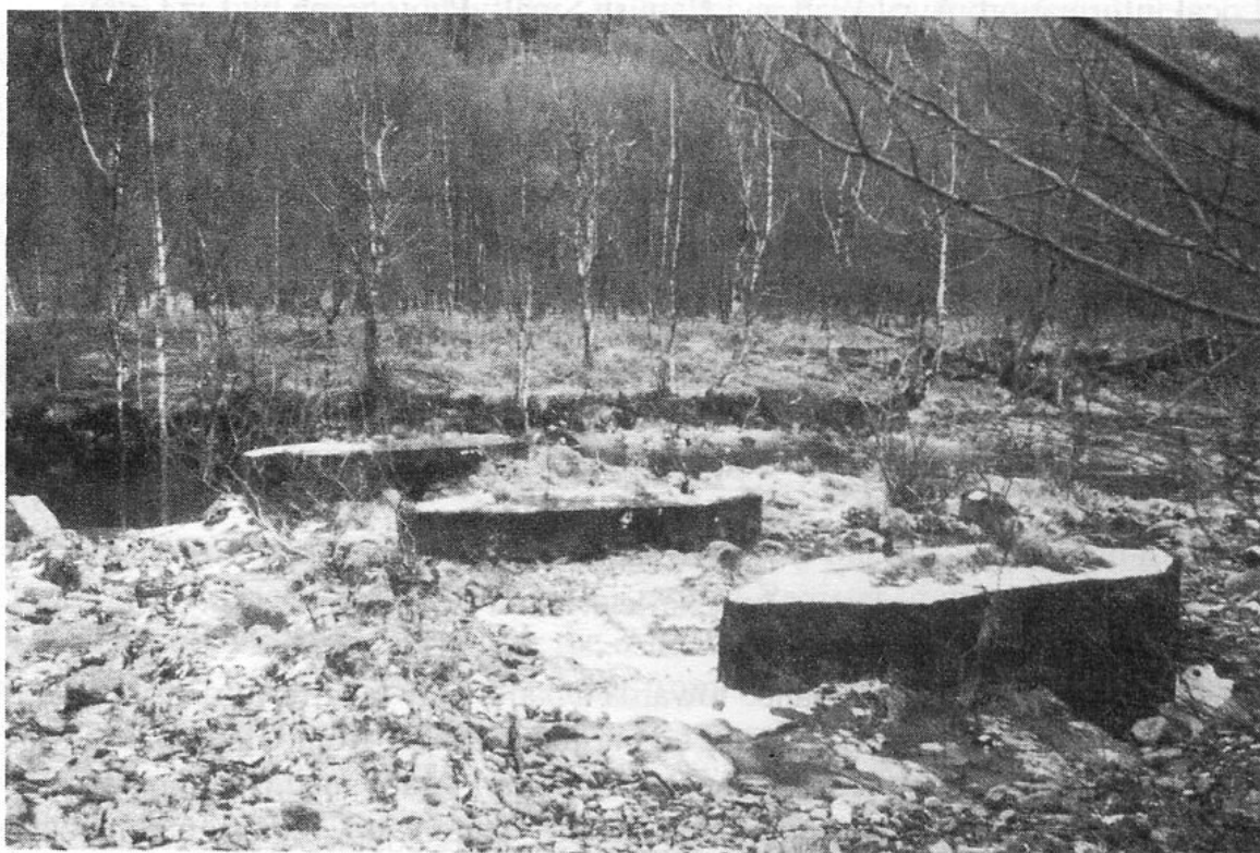
The remains of the bridge across to the camp
