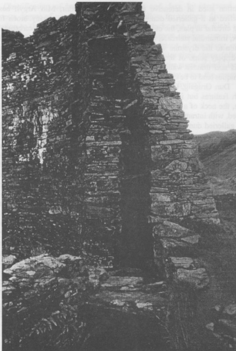
Dun Telve, Glenelg. Note the variety of stone used in the wall and the slabs tying the walls together. Photo: R. Harvey
