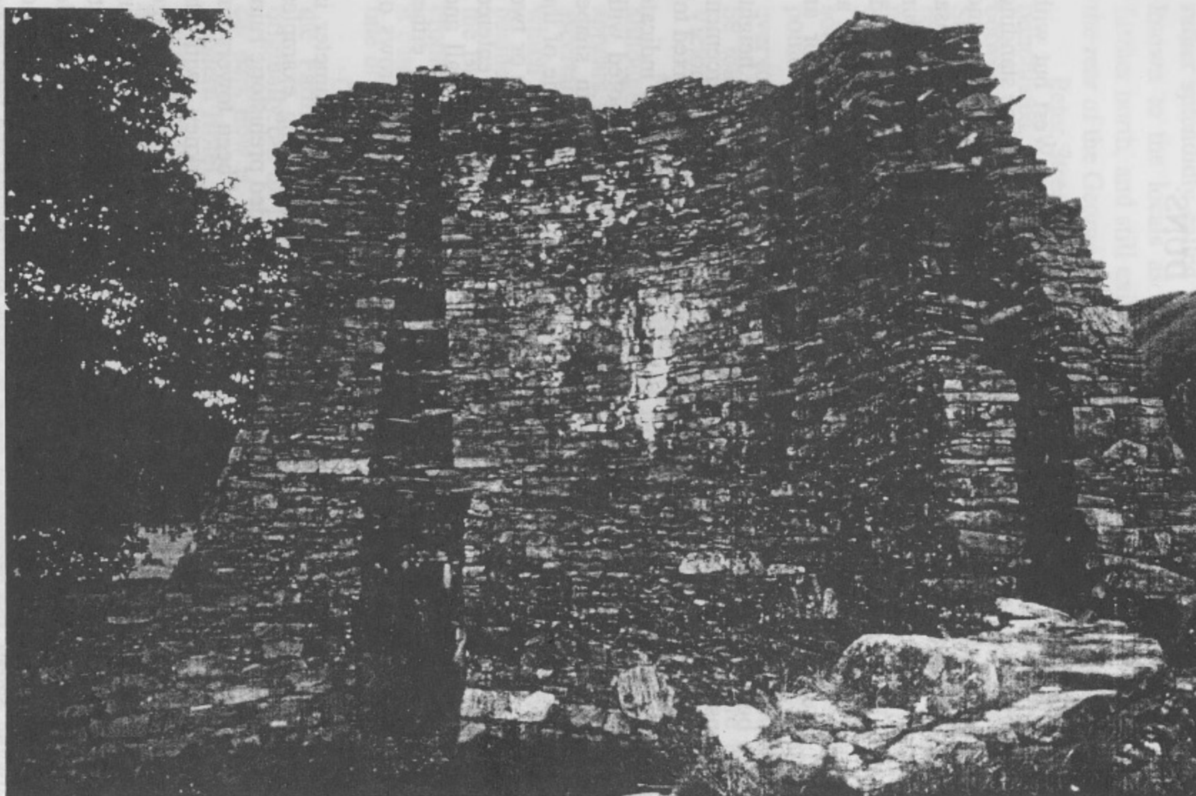
Dun Telve, Glenelg. The entrance is on the left with a recess in the wall to one side that has been interpreted as a possible guard cell. Note spaces in the wall above the entrance and elsewhere, perhaps to lighten the load on the doorway lintel and/or provide added ventilation. Photo: R. Harvey
